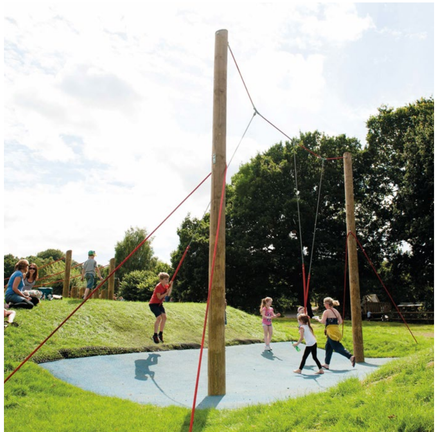
The photo shows different tensioning ropes, Photo © Paul Upward
