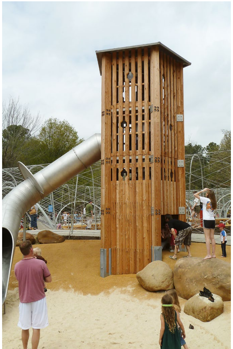
This picture shows a special version of the Middle Pentagonal Tower, closed to a height of 2.40 m.
